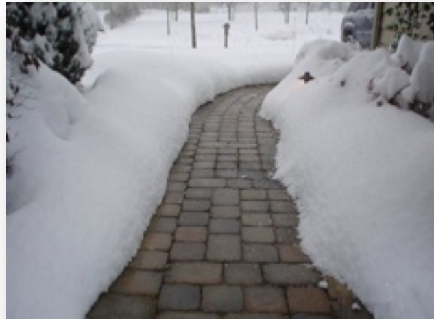
Photo courtesy of Ken Baker, K energy
